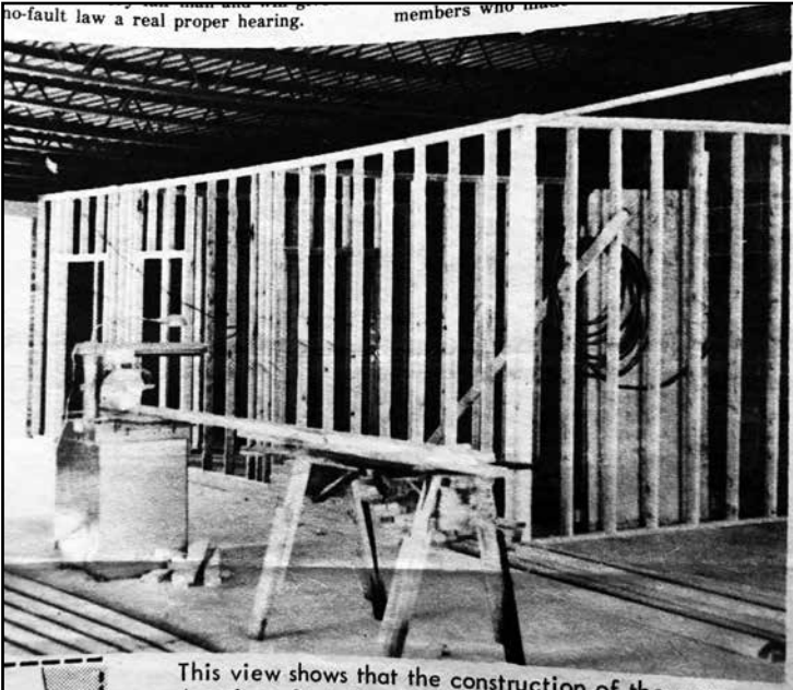
This view shows that the construction of the new American State Bank of Grygla is now progressing in-doors.
