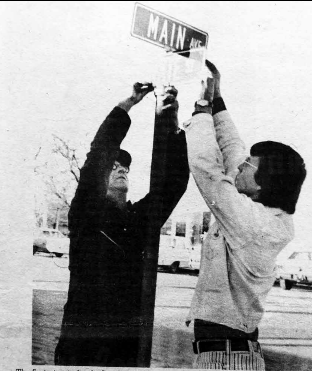
The first street sign in Grygla is being put up by Thorfin Ostby and Jim Houg on the corner of State Street and Main Ave. by the bank building. A total of eight streets signs will be installed.
