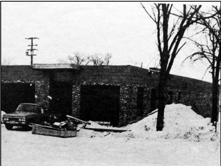
Bank Construction Progresses - The progress on the new bank in Grygla has made rapid progress in the past week. Now the glass windows have been installed and work is progressing on the fixtures for the bank. March 3rd might be the day the new bank will open if construction continues to go well.
