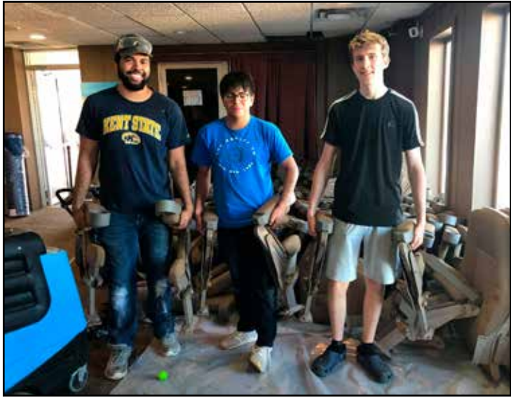
Jeff says about eight people are working on the renovation at Falls Cinema, including these younger employees. L-R: Caleb Richardson, Noah Grove and Trian Petrescue were busy hauling out old seating.
