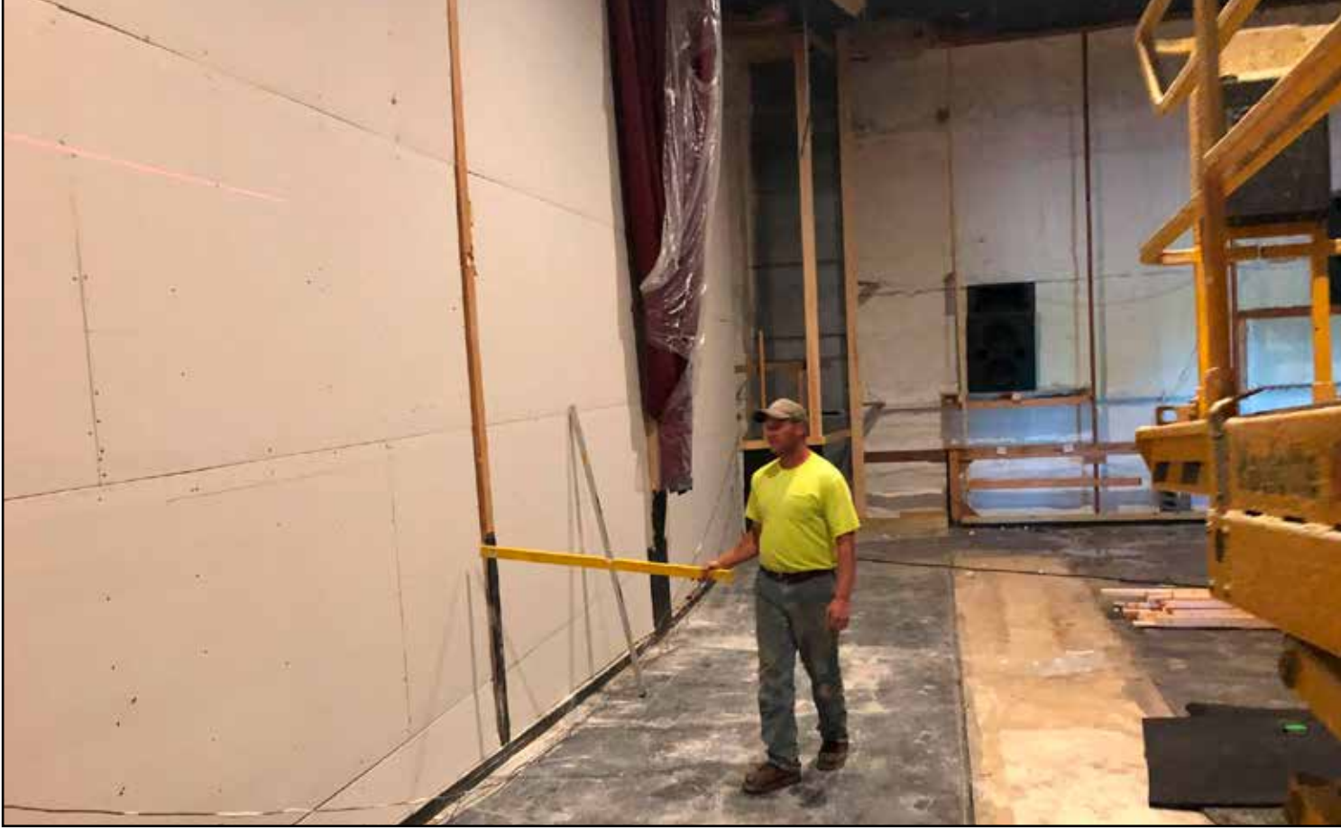
Jeff and Parker were busy drawing out where the platforms would be built. The new luxury loungers are being made down in South Carolina and will be installed on the platforms. Photos by Grygla Eagle Newspaper
