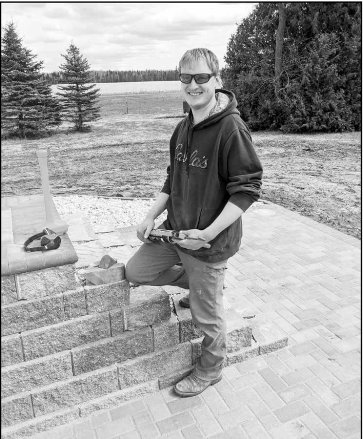
Tyler Aune is pictured gluing bullnose caps onto new entrance steps. The other pictures are examples of his work. Photos courtesy of Alyssa Aune
