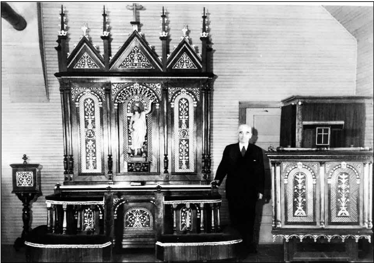
(1938) Bethel Lutheran Church in Grygla. Altar, pulpit, kneeling rail and baptismal font built by John Franzman. This altar is now at the Historical Society in Warren, MN. This was the second creation John made for Bethel, sending the original and smaller one to a church in Goodridge.
