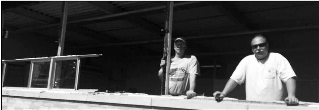
You'll need to take a drive by the Grygla School if you haven't seen the new windows being installed. The east side of the building is getting a window upgrade and it should be completed within a week. Along with 3-6 grade, the music room also had new windows installed. Pictured is Jim Smeby and Bill Neuschwander. (Lowell Smeby is also helping with the project, but was not pictured.) Photos of completed project coming soon!
