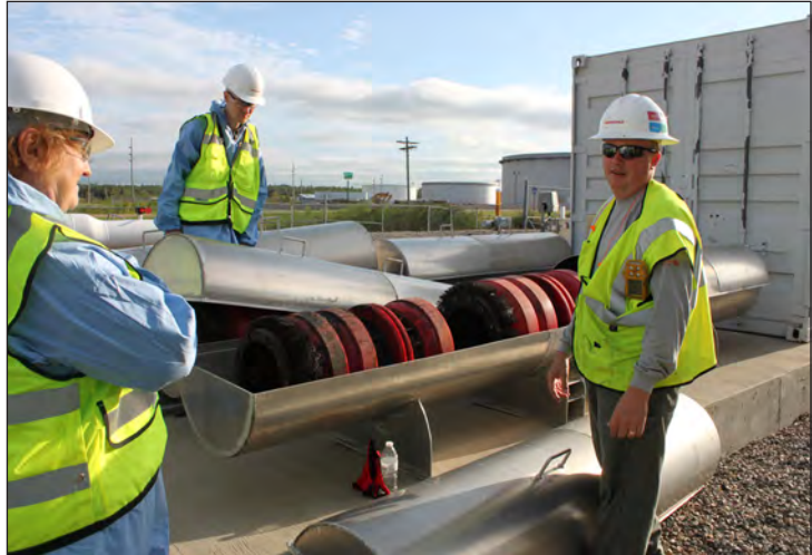
The apparatus in this container is called a pig. These are inserted into the oil pipelines to perform various maintenance operations. It can be used for cleaning or inspecting of the lines. It can be done without stopping the flow of the product that is being sent through the line.
