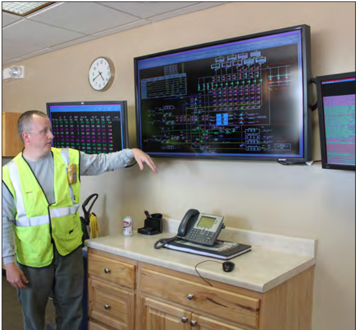
Bill Palmer, Enbridge Terminal Supervisor at Clearbrook explained the control system. They check levels, tanks, volume and where the oil is going. Various products are kept in separate tanks and they can all be monitored with this system. Monitoring is constantly being done by sensors that transmit data to Enbridge's central control facility in Edmonton, Alberta.
