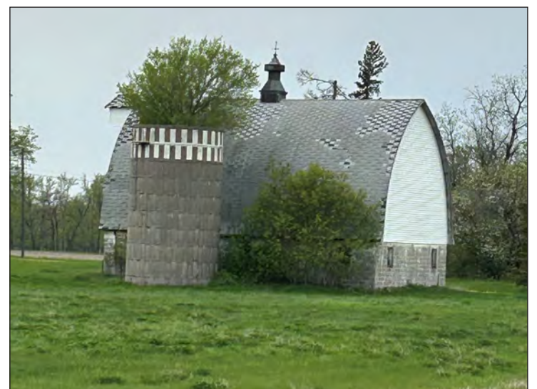
This picture was sent to me. The barn shown is cement on the bottom with a wooden hayloft on top. Notice the tree growing out the top of the silo. I believe the barn is located west of Mahanomen, MN.
