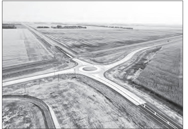
Hwy 75 roundabout north of Crookston: The project was led by Polk County to improve safety the Highway 75/County Road 21 intersection north of Crookston.
