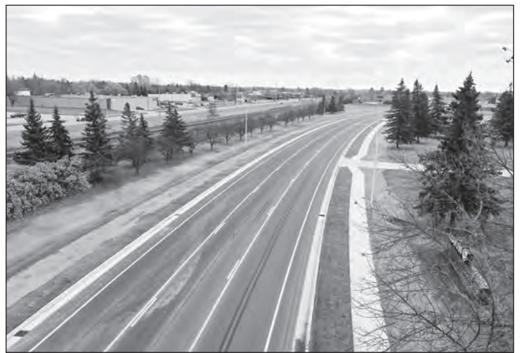
Hwy 11 Warroad: Completed year one of a three-year project that will reconstruct or resurface Highways 11 and 313 through Warroad and improve safety and access. Crews will return in 2025 to complete the roundabout at Highway 11/313 and begin Highway 11 bridge construction.
