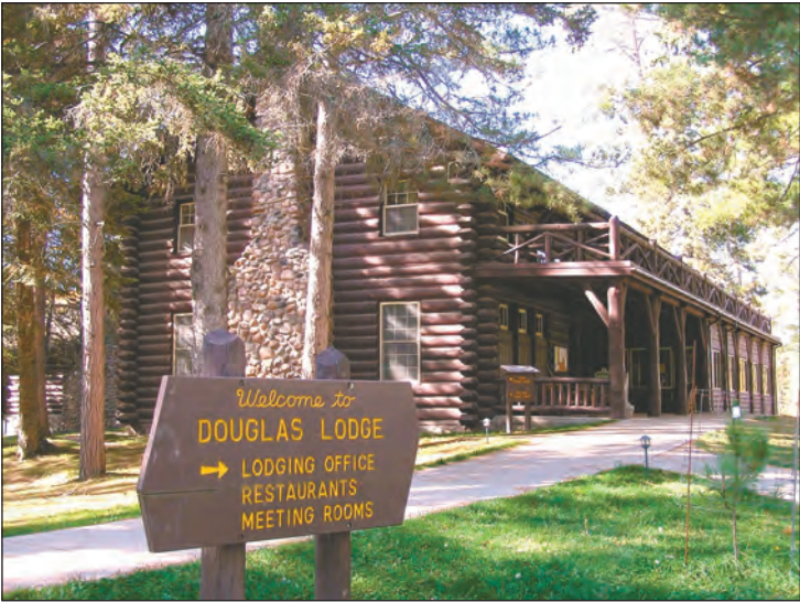
Douglas Lodge: The top priorities in the park's 20-year water and sewer line rehabilitation plan include: The north and south water and sewer lines that serve historic Douglas Lodge. The building is 110 years old, the infrastructure is estimated to be at least 40 to 50 years old. Also needing work is the Bear Paw campground water and sewer lines, as well as the water and sewer lines that feed the park's cabins. Nicollet Court: Funding is needed to design and begin rehab of the historic 88-year old Nicollet Court, currently not open to the public, so that it can become a rental facility.
