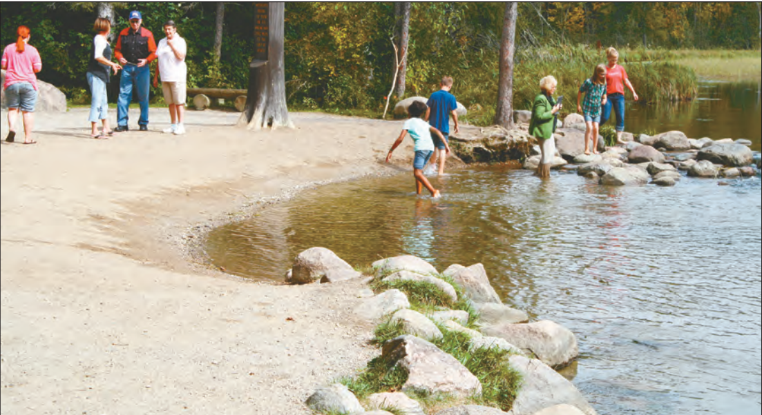
There is a need to repair serious erosion at the Headwaters of the Mississippi River, caused by the large number of visitors received each year.
