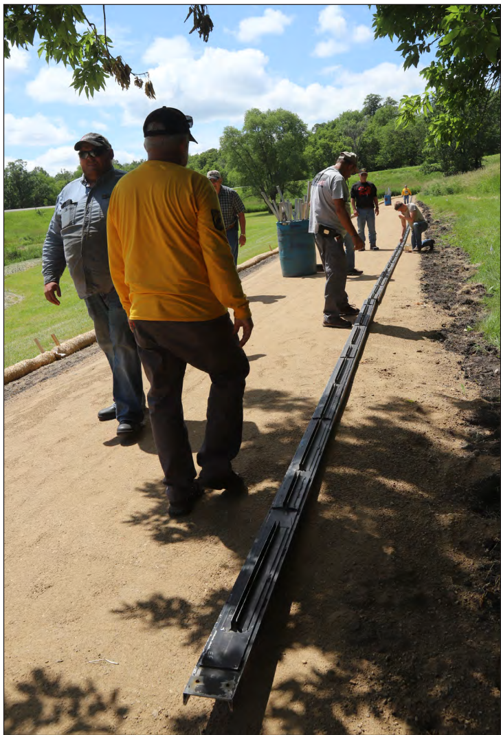
Lining up the rails for the Vietnam Wall.
