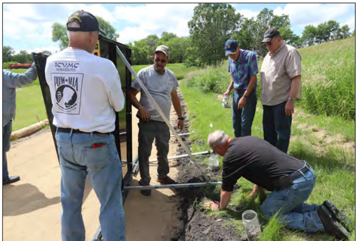
Getting the stakes down to stabilize the Wall.
