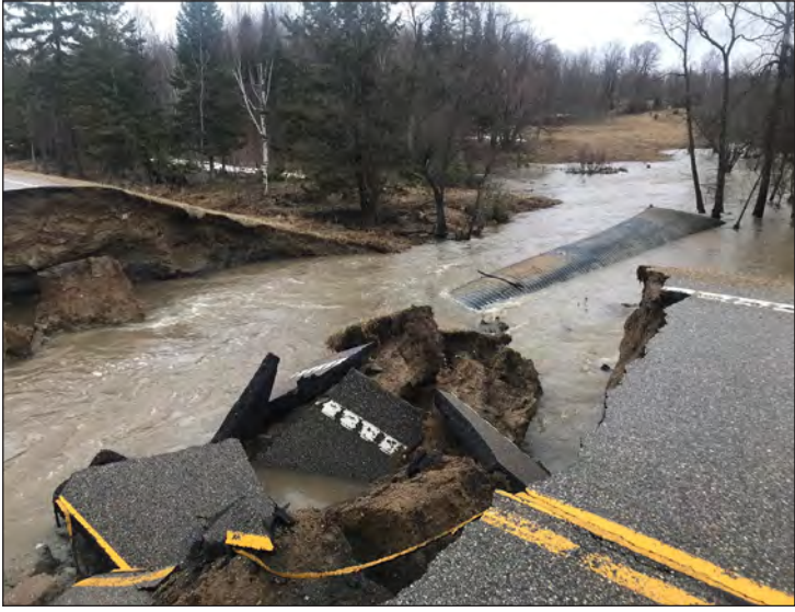
Above, Clearwater Lake Road by Spike Lake... about 50 feet of road completely gone, west of Bev Charles driveway. Below, east of her driveway on the Spike Lake side, ditch is completely washed away. Photos by Bruce Emmel.
