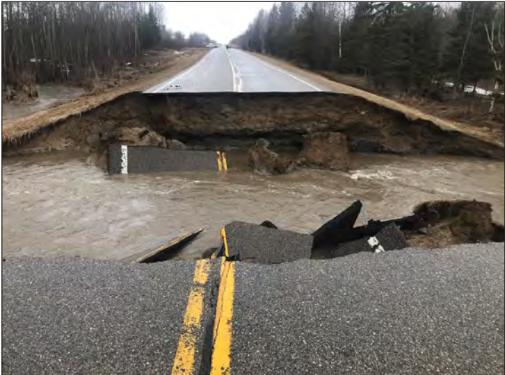
Above, Clearwater Lake Road by Spike Lake... about 50 feet of road completely gone, west of Bev Charles driveway. Below, east of her driveway on the Spike Lake side, ditch is completely washed away. Photos by Bruce Emmel.
