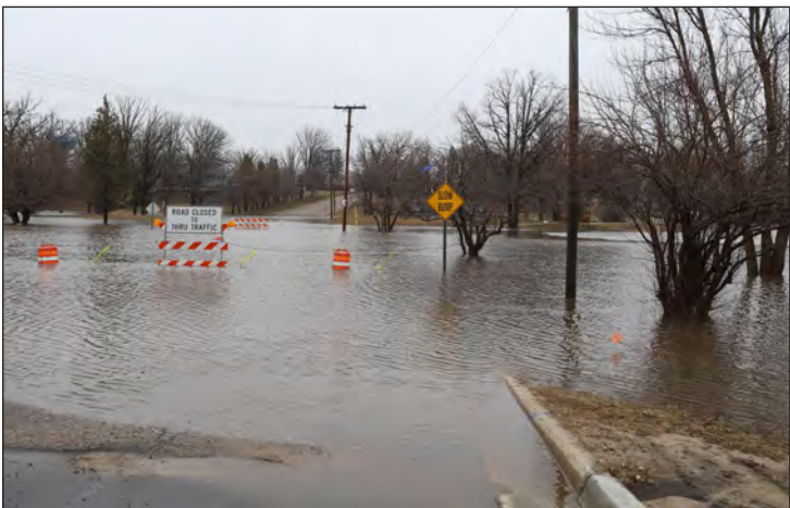
The water over the dam north of the Clearbrook Elevator. Photo by Leader-Record.
