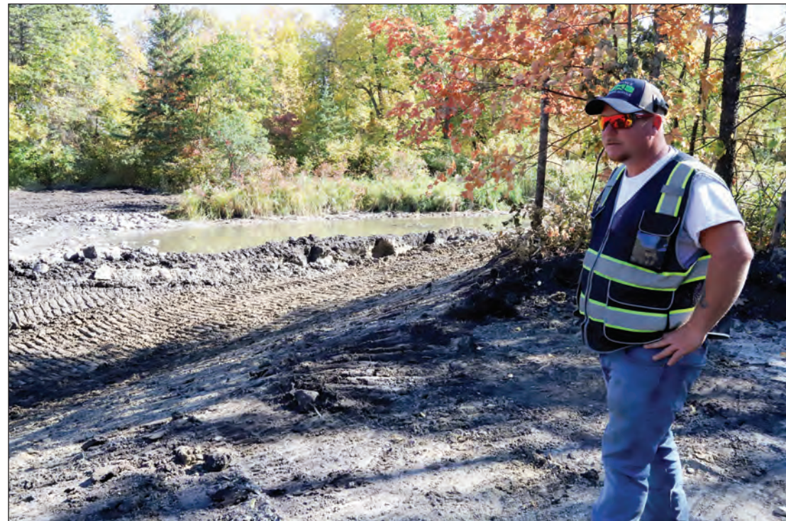
Getting the water diverted so that the cement work can be done on the dam.
