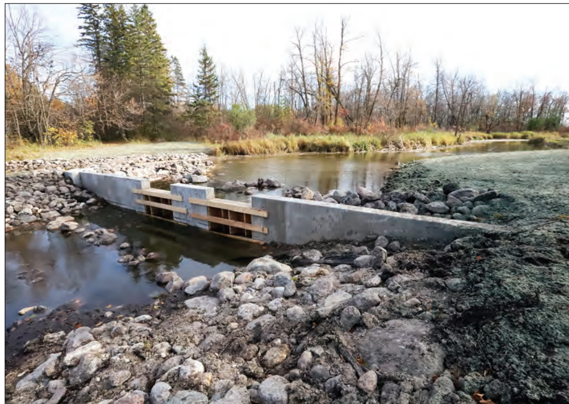
Getting the water heading in the correct direction. The lifts in place with water at two different levels. Davidson Construction Company of Newfolden did the work this year.
