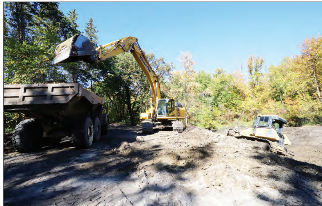
Starting to get the dirt moved to make way for the Pine Lake dam project.
