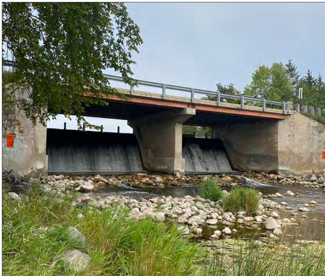
The dam at Clearwater Lake now has water coming over the spillway. With the weather this summer it has been a lot lower from the dam down the river.
