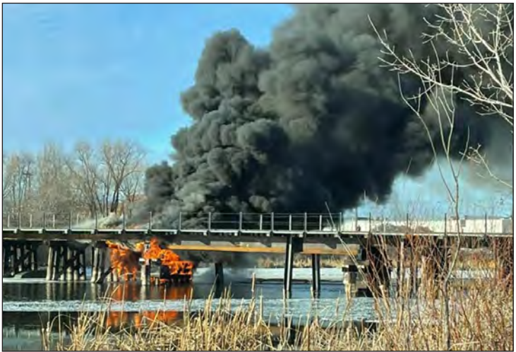
A fire caused "moderate damage" to a BNSF railroad bridge on Monday afternoon in Bemidji. (Bemidji Fire Department photo)
