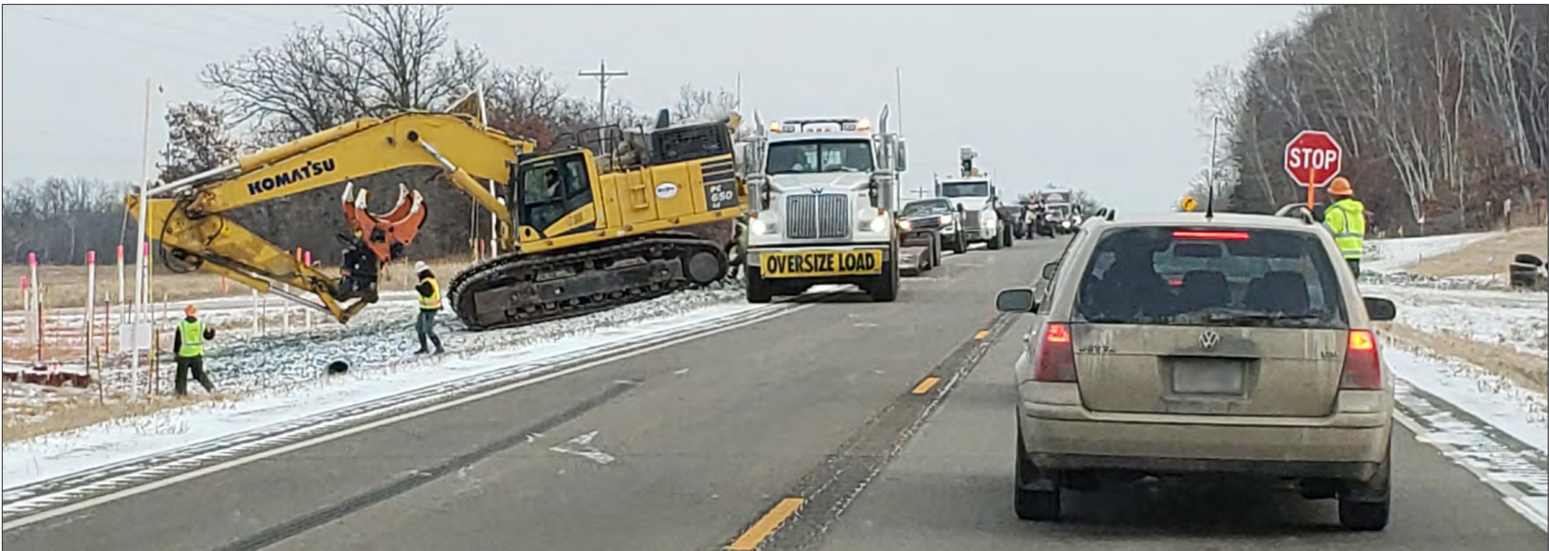
If you're driving around the Trail - Gully area you will notice there is lots of activity along the pipeline route. Last Wednesday, Enbridge crew members were unloading large equipment just east of Trail.
