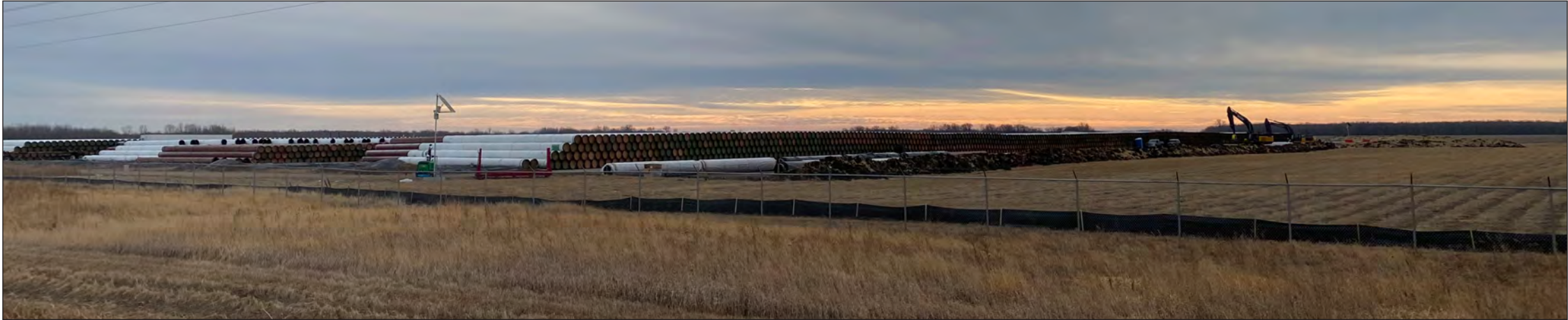
Acres of Pipeline Pipe are in position (east of Plummer) for distribution when needed for the Line 3 project.
