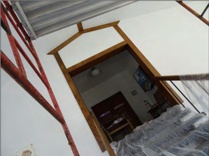
New trim dresses up the entry at Lund Church in Gully while helping to conceal patches on troublesome, reoccurring cracks in the plaster.
