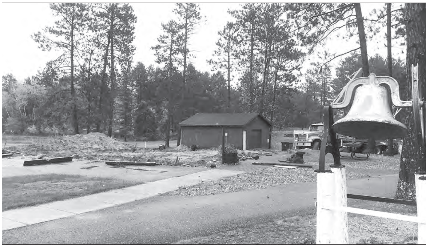
There will be a new clubhouse at the Twin Pines golf course next season. The old one is gone with Darren Lindgren of Bagley taking it down. The new one is under construction with contractor Duane Lewis of Universal Builders. Tom Riewer, the golf course director stated that the new one will be 52 x 32 feet and will also have a 12 x 42 foot attached screen porch.
