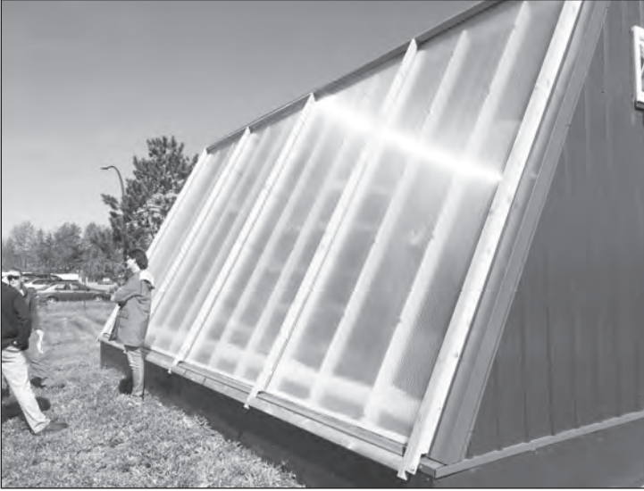
Triple pane polycarbonate panels do a good job to let in the warmth and keep it in!
