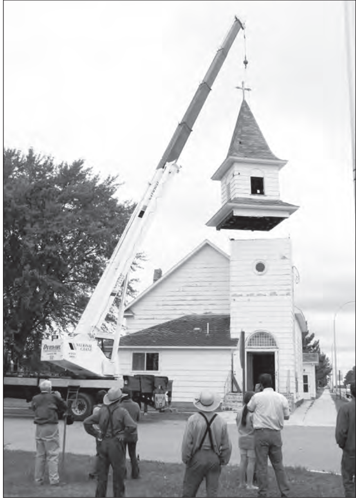
The steeple was carefully lifted off the top of the Salem Lutheran Church before making its way to its new home at the Norris Syverson farm.
