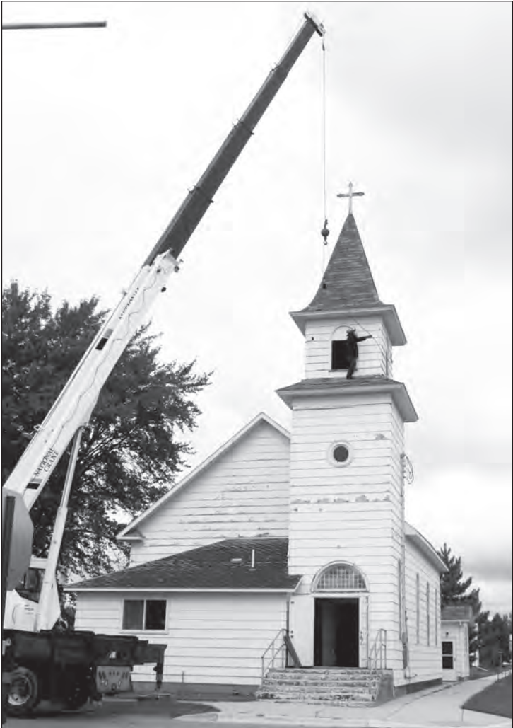
A worker balances himself on the edge of the steeple as they prepare to lift it off of the Salem Lutheran Church.
