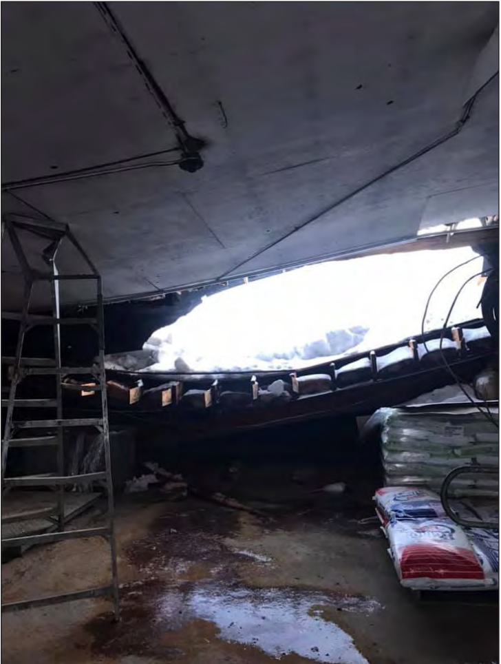
The shop building at the McIntosh elevator had it's roof collapse in early March due to the incredible snow load that was part of many buildings having roof collapses or buildings falling under the heavy weight.
