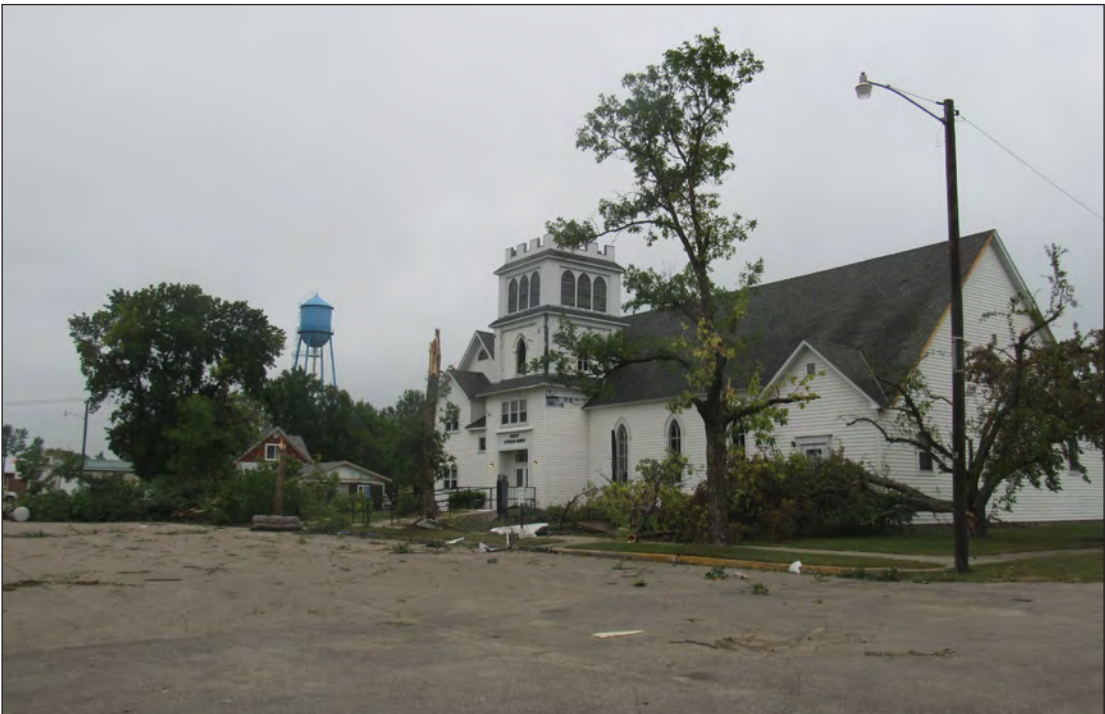
A late night storm that hit NW Minnesota Sunday night did considerable damage in Winger. Calvary Lutheran Church had severe damage.
