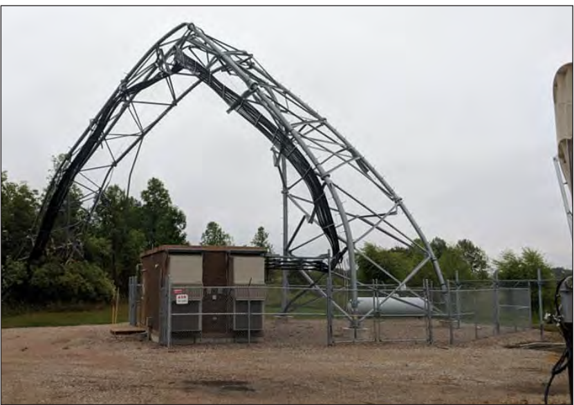
Last night, August 26th, 2018, an apparent tornado touched down at the City of Fosston's cable TV east of Fosston on the Columbia road. The Verizon cell tower that was a self supporting tower twisted and buckled. Fosston cable subscribers received channel 12 from that tower. The antennas that receive all of their other local channels were also destroyed as well as two large satellite dishes that receive numerous other channels. It will take some time to get everything restored while they wait for new dishes to arrive and be assembled. Photo by Jim Offerdahl, Mayor at City of Fosston and Chief Engineer at Offerdahl Broadcast Service, Inc.
