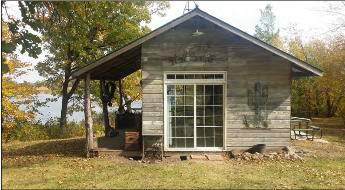
The cabin, on a lake in Erskine, Minn., started as an area for outdoor cooking.
