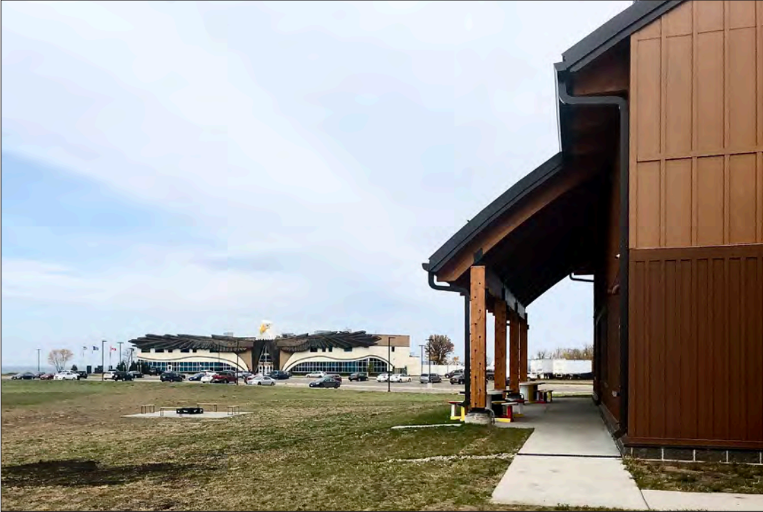
Looking toward Tribal HQ and the Lake beyond. In the foreground is a Fire Ring and lounge/picnic area outside the Center.
